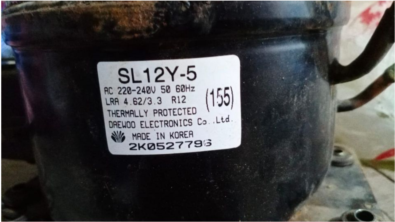
Mbsm.pro, SL12y-5, Daewoo, Refrigeration ,Compressor, 1/10 HP, 220v 60hz, R12
