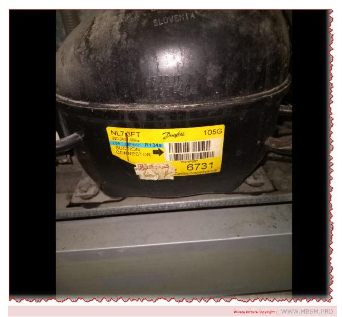
the 105G6731 is a model number for a tropical compressor manufactured by Secop,
