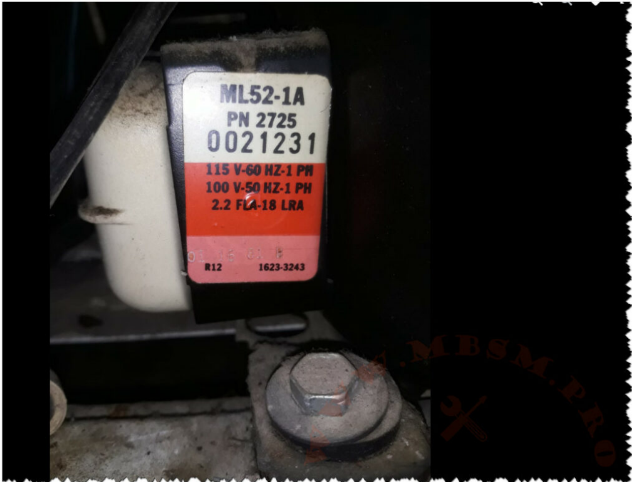
Mbsm.pro, Compressor, ML52-1A, PN 2725, r12, QB66C13GAX5, 1/5 hp, r134a, freezer, 6 raks
