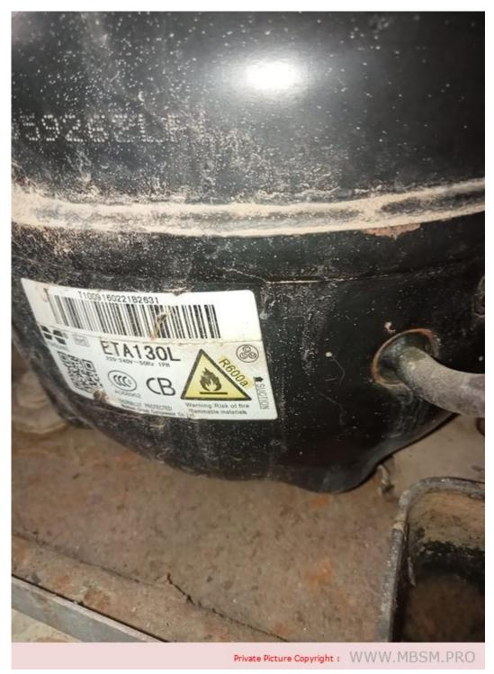
Mbsm.pro, compressor, Huaguang, R600a, ETA110L, 1/5 hp, ETA115L, 1/4 hp, ETA130L, 1/4 hp++, ETA150L, 1/3 hp
