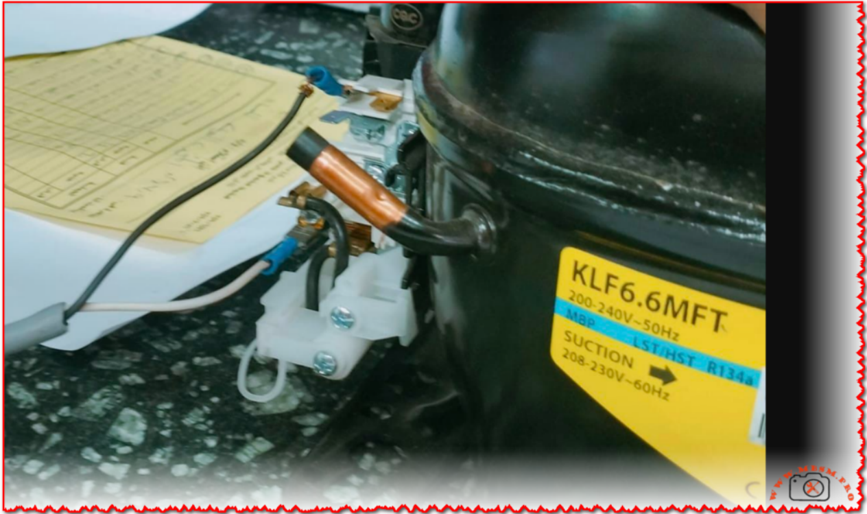
Mbsm.pro, Compressor, KLF6.6MFT, KLF66MFT, 1/5hp , mhbp, Big++, 187 w, Secop, R134a
