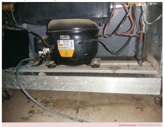
Mbsm.pro, Compressor, hpk190A, 1/4 hp++, 1/3 hp-,R600,HMBP, 220/240V, 50Hz, 12.11 cc , unionaire, UR-350, 340 L, R600a/48g, 0.87 A
