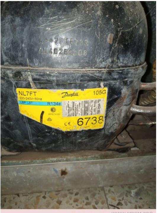
Mbsm.pro, Compressor, 1/5 Hp, NL7FT, SECOP, DANFOSS,105G6728, 105G6738, Lbp, r134a
