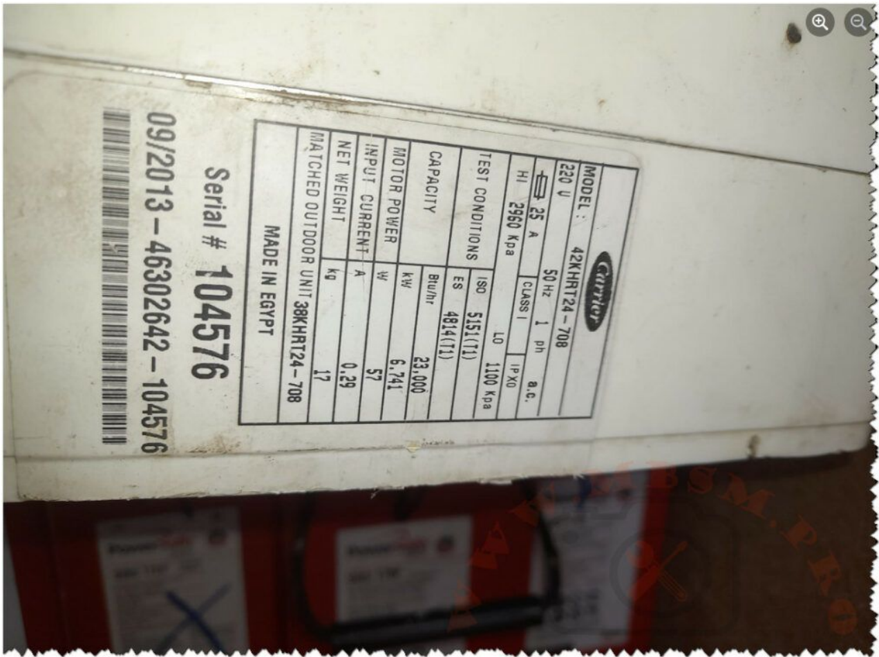
Private Picture Copyright : WWW.MBSM.PRO Mbsm.pro, air conditioner, 42khrt24, 24000 btu, 2 t, 3 hp, r22
