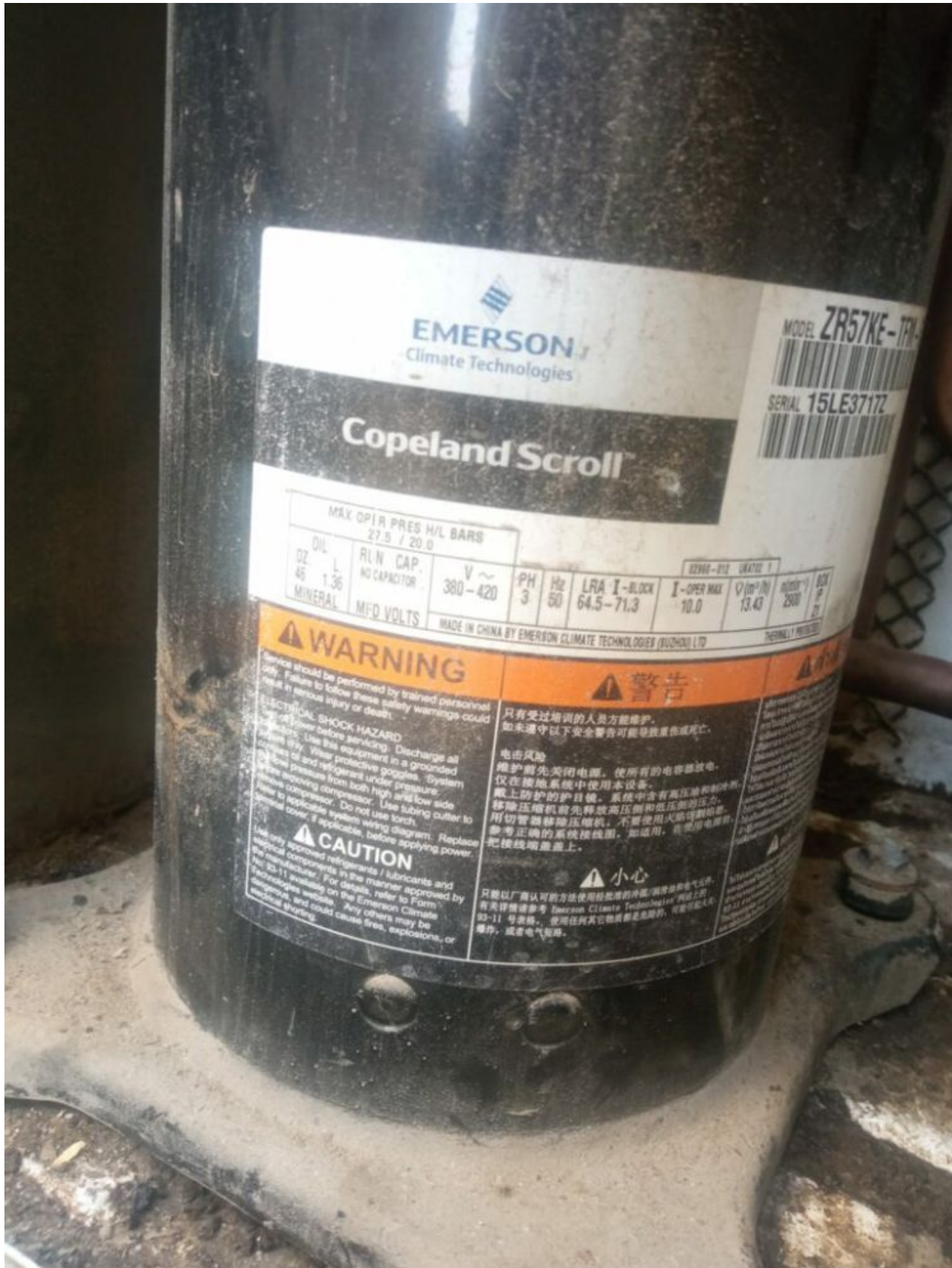
Mbsm.pro, compressor, ZR57KE-TFD, 4.8 hp, 13.900 w, 47500 btu, r22, emerson, copeland, scroll, ZR Series, 380-420V/50Hz, 3 Ph
