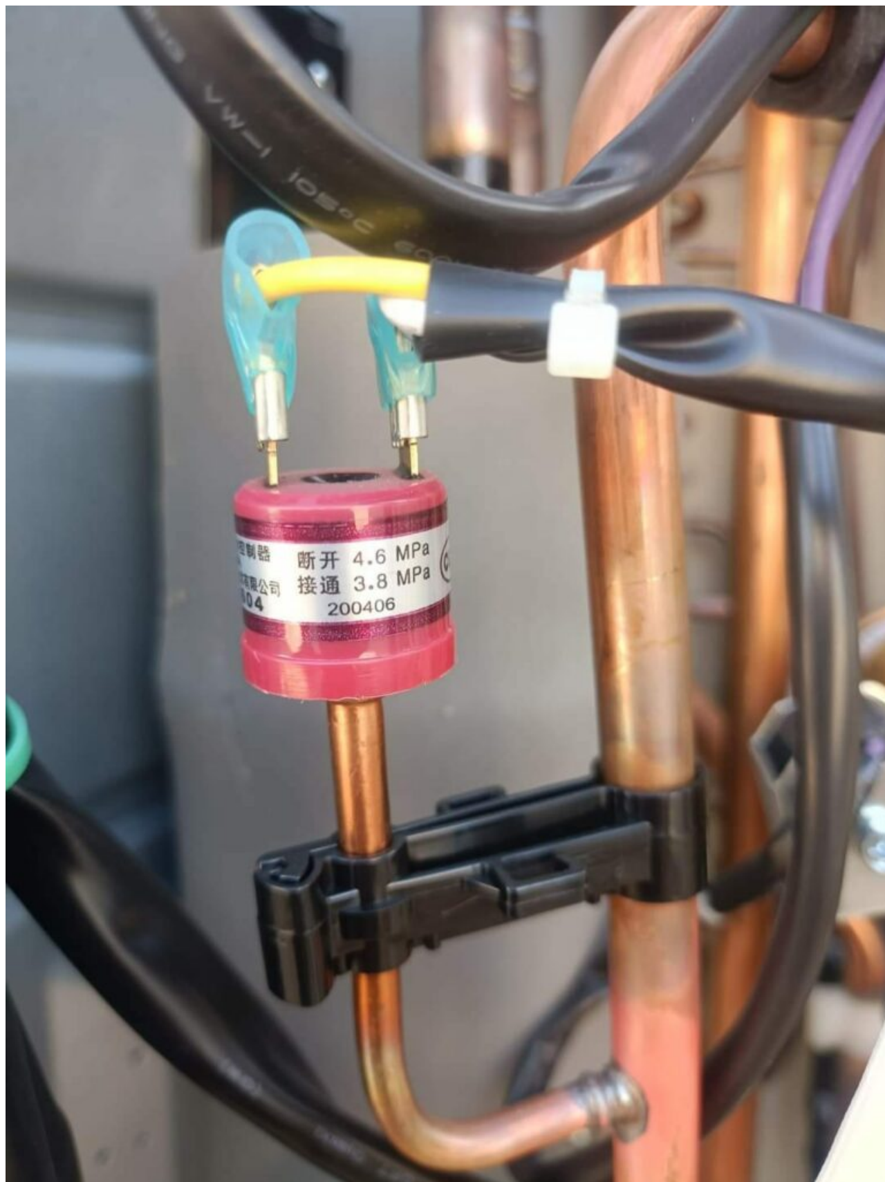
low-pressure cut-off switch
