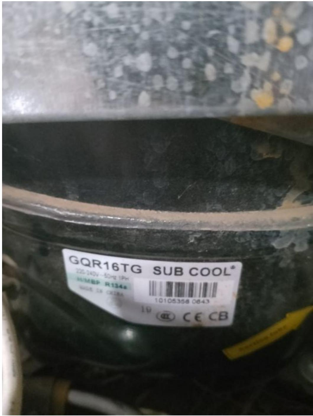
GQR16TG, light, commercial, refrigeration, compressor ,1 / 2+ HP, 220V/50Hz,
