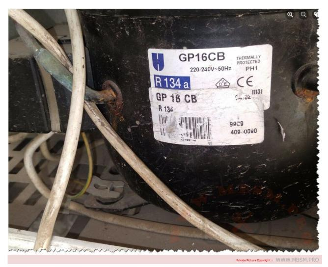
Mbsm.pro, Compressor, Cubigel, GP16CB, R134A, LBP, 3/8 hp
