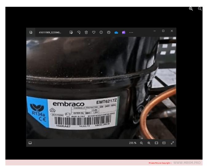
Mbsm.pro, Compressor, Embraco, Emt6217z, NT6217Z, 3/4 hp, hbp, r134a
