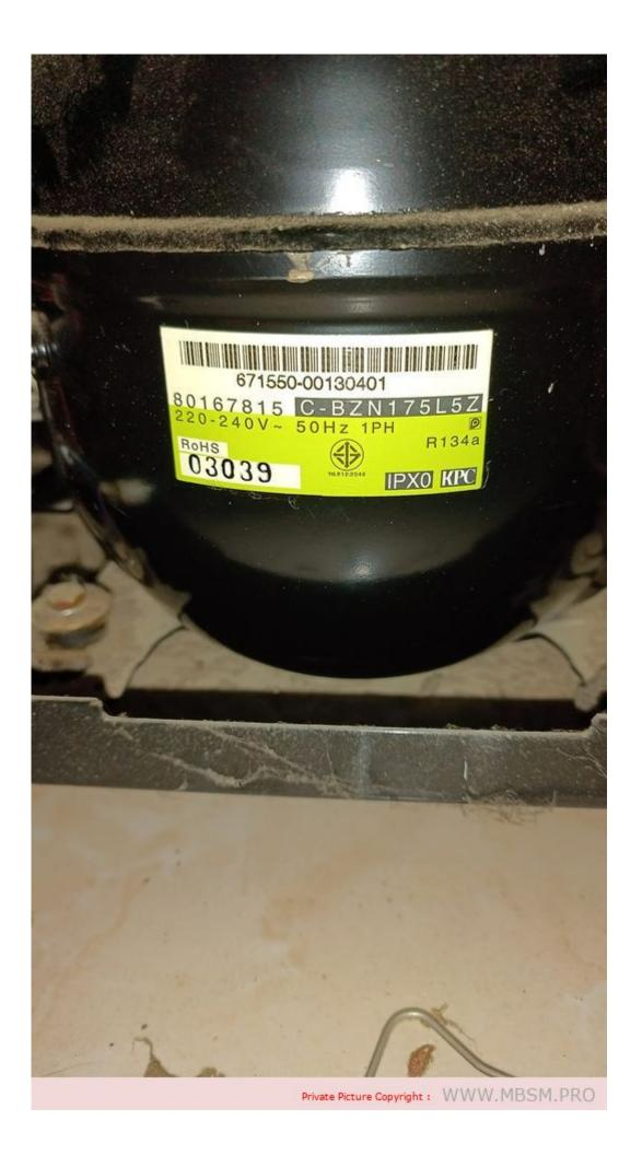
Mbsm.pro, Compressor, C-BZN175L5Z, KULTHORN, piston, refrigeration compressor, 1/5 hp
