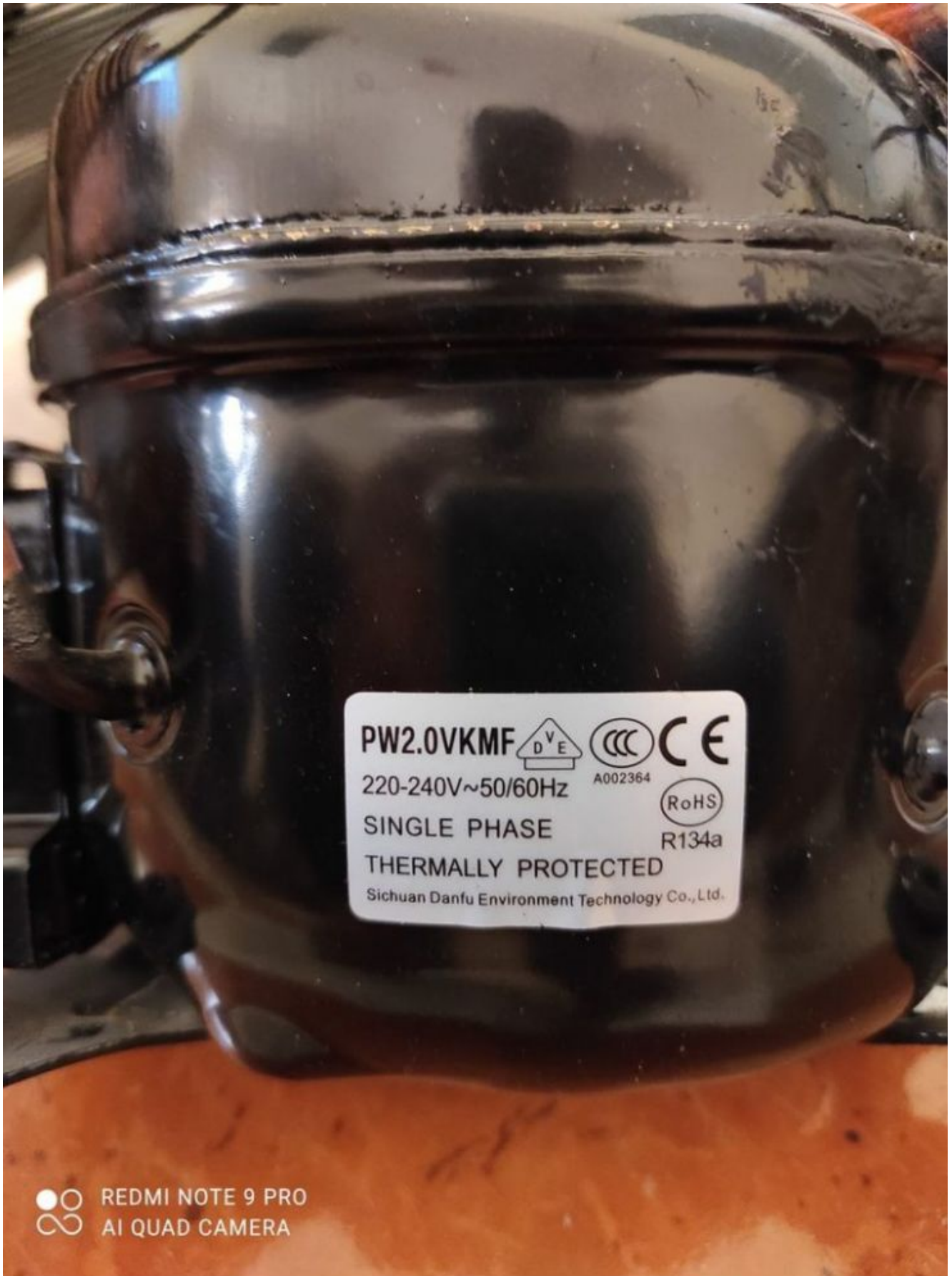
R134A, LBP, Motor, Danfu, Compressor , PW2.0VK, 1/15hp
