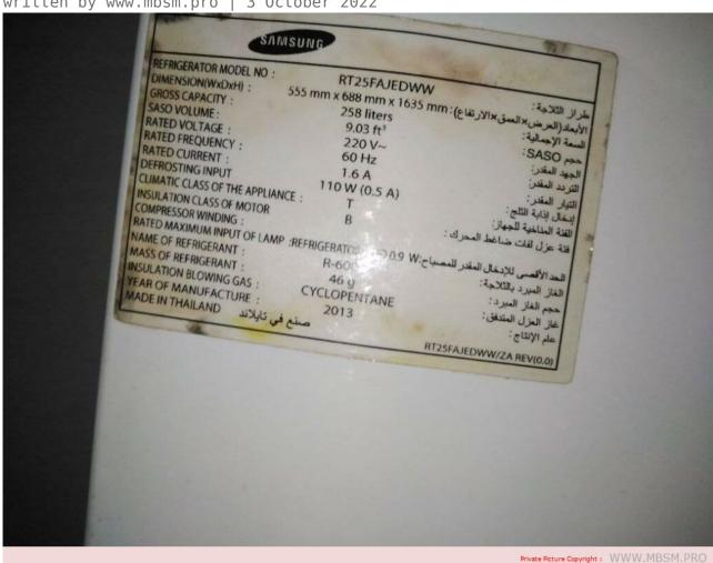
Mbsm.pro, Refrigerator, RT25fajedww, 250 L, no frost, inverter, Compressor, BDC, 1/6 hp, lbp, R600a, 46g, 220v
