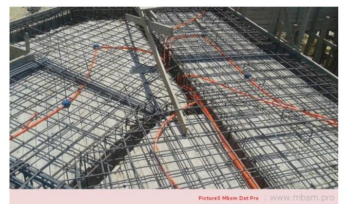
Mbsm.pro,The risk of extending the electric hoses under the reinforcing steel for ceilings
