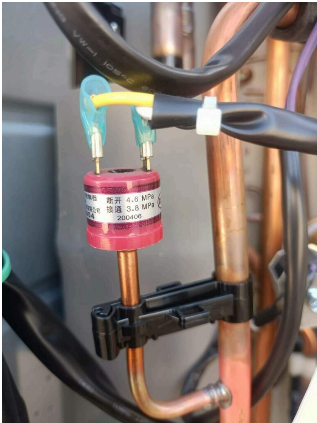
low-pressure cut-off switch
