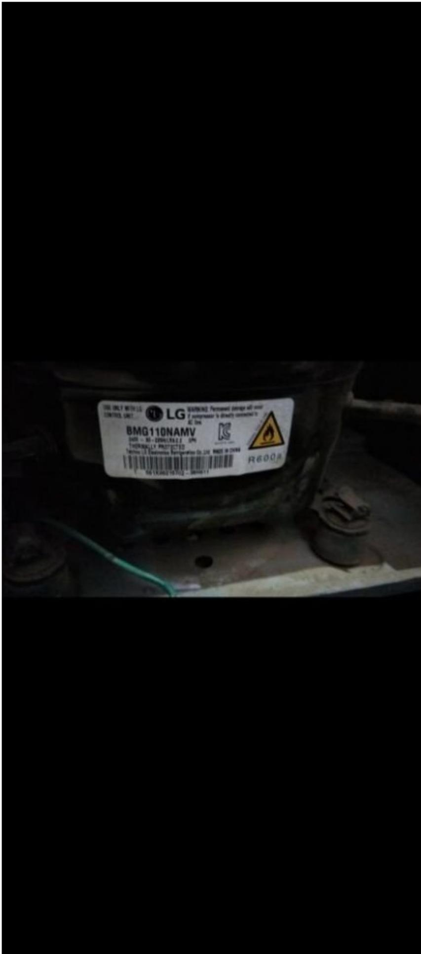
Mbsm.pro, Compressor, inverter, LG Refrigerator, BMG110NHMV, BMG/BMA LG, Lbp, 1/4 Hp , R600A
