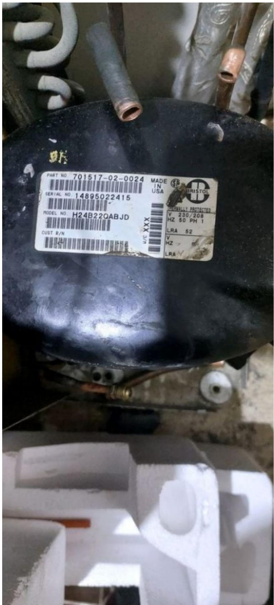
Mbsm.pro, Bristol, Compressor, H24B22QABJC, 21800 btu/h, H24BQ SERIES, 6397 W, 230 v, 1 Phase, lra 52 A, Compressors, Chillers & Condensers, high temperature, R22, basic model, model B, PSC capacitor, line break internal, capillarie, 0.64/80 cm, 0.70/100 cm
