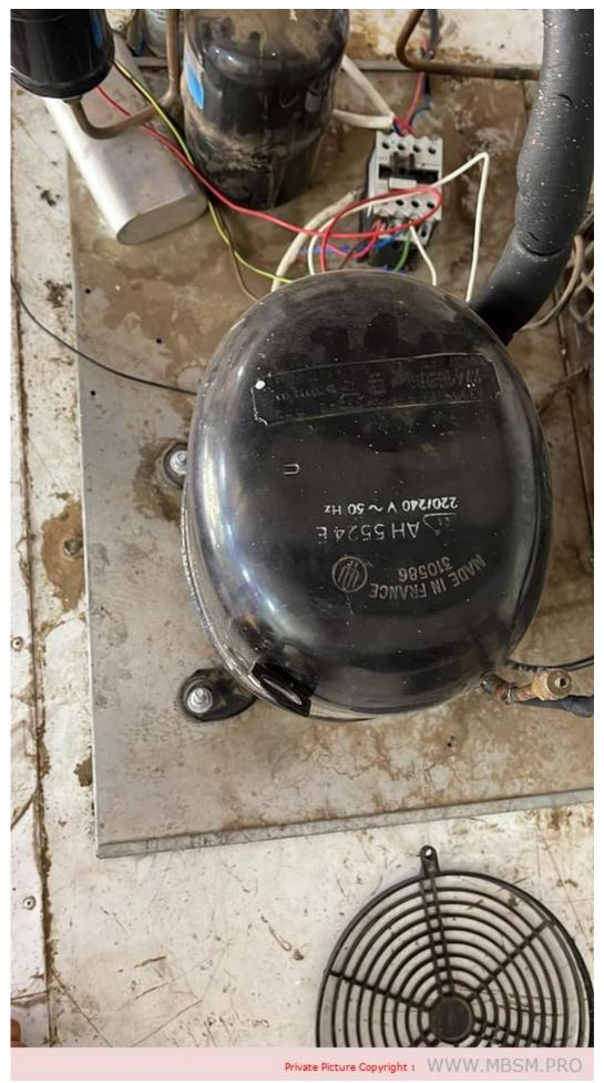
Tecumseh, AH141FT-014, R22, FH5524E, AH5524E, 2HP/, 2Ton, 208-230V 60Hz, 1Ph,
