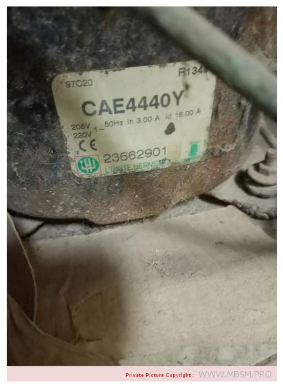
Mbsm.pro, COMPRESSOR, 1/3 HP ++ (big), HERMETIC, TECUMSEH, CAE4440Y, AE4440Y, HBP, R134a, 220-240V, 50 Hz, 1 PH, CSIR
