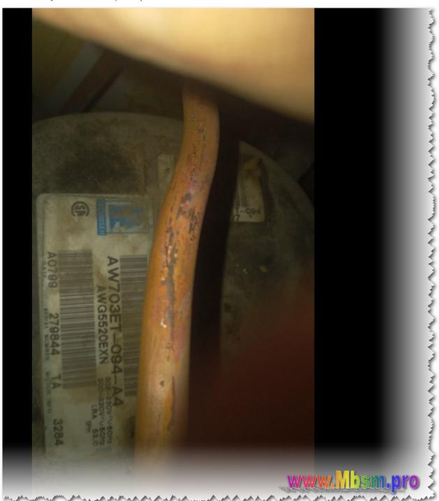
The AW703ET-094-A4 is a model of compressor produced by Tecumseh, specifically designed for air conditioning and high back pressure (HBP) applications. Here are the key specifications:
