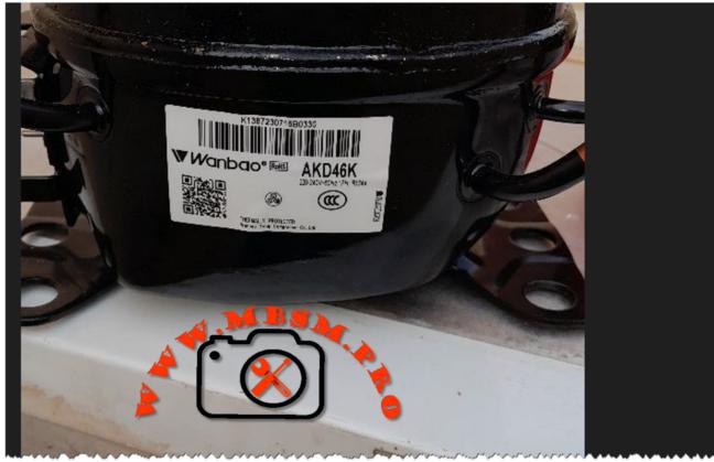
Wanbao AKD46K compressor. This compressor is used in refrigeration systems and is associated with specifications like R-134, 23.3C, and 115W. It is a part of the Wanbao (Huaguang) compressor series, which includes models like ATA55K,
